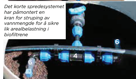
Spredesystem i liten biofilterkum
