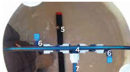
Spredesystem i stor biofilterkum
